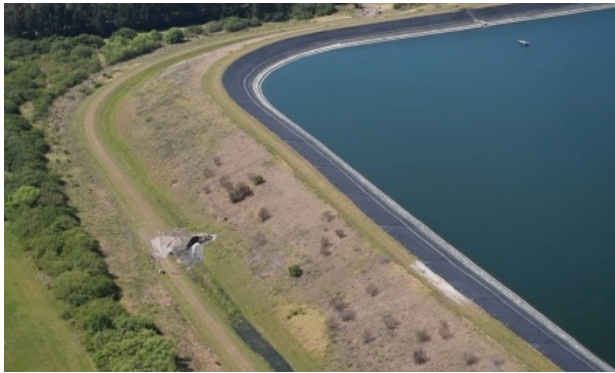
Drone shot of the leak
